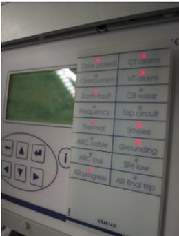
Figure 1 VAM 16 D external LED panel as a part of the feeder/motor manager VAMP 255
